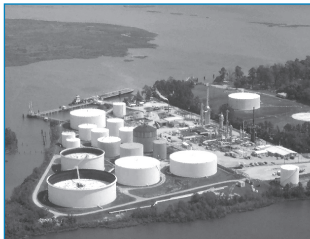
BULK PLANT OR TERMINAL. 515.1 DEFINES SUCH A PLANT AS A LOCATION “WHERE FLAMMABLE LIQUIDS ARE RECEIVED AND ARE STORED OR BLENDED IN BULK FOR THE PURPOSE OF DISTRIBUTING SUCH LIQUIDS BY TANK VESSEL,” ETC.
