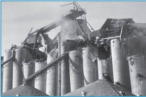
ELIMINATING DISASTERS LIKE THIS REQUIRES CAREFUL CLASSIFICATION OF AREAS AND THE USE OF THE PROPER ELECTRICAL EQUIPMENT.
