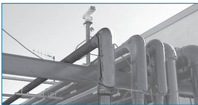
TYPICAL CLASS I, DIVISION 2 RIGID CONDUIT INSTALLATION.
